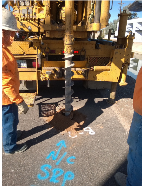
Photo 2 – Auger Drilling at Boring B-8
